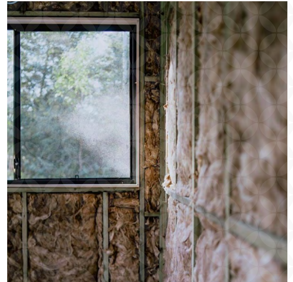
FIGURE 11 Insulation in stud walls SOURCE: Earthwool
