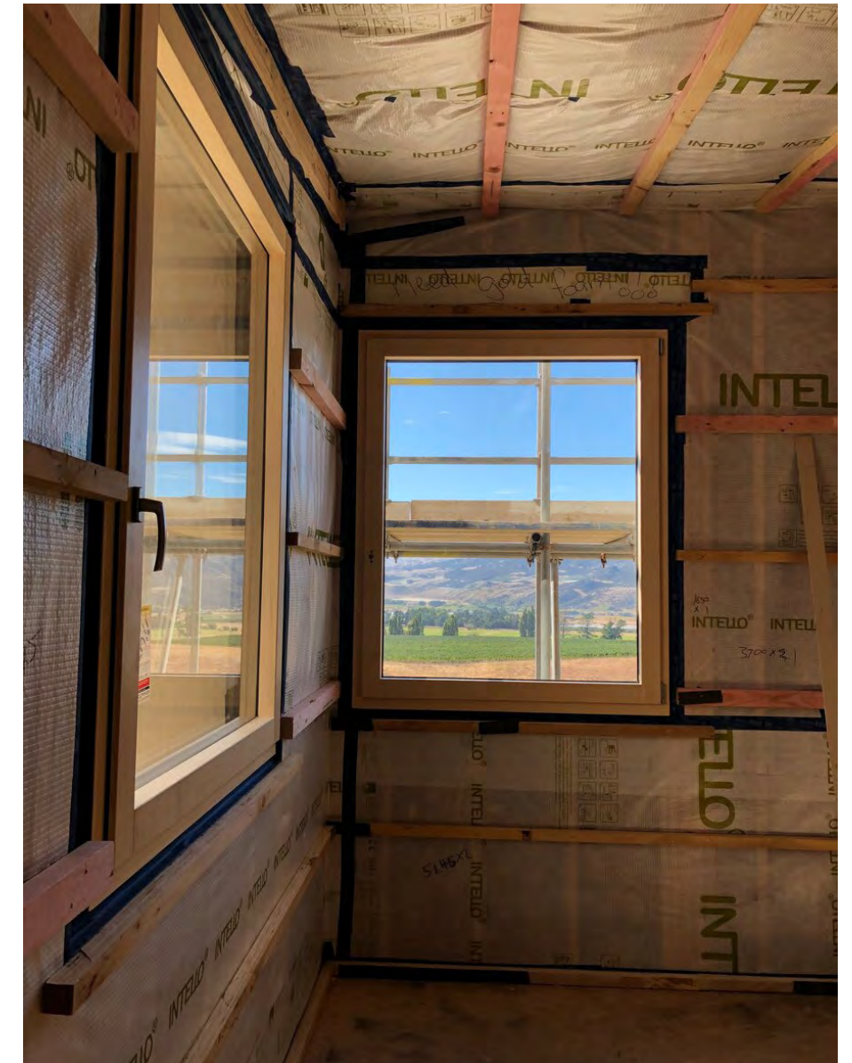
FIGURE 17 External wall wrap SOURCE: Team Green Architects
