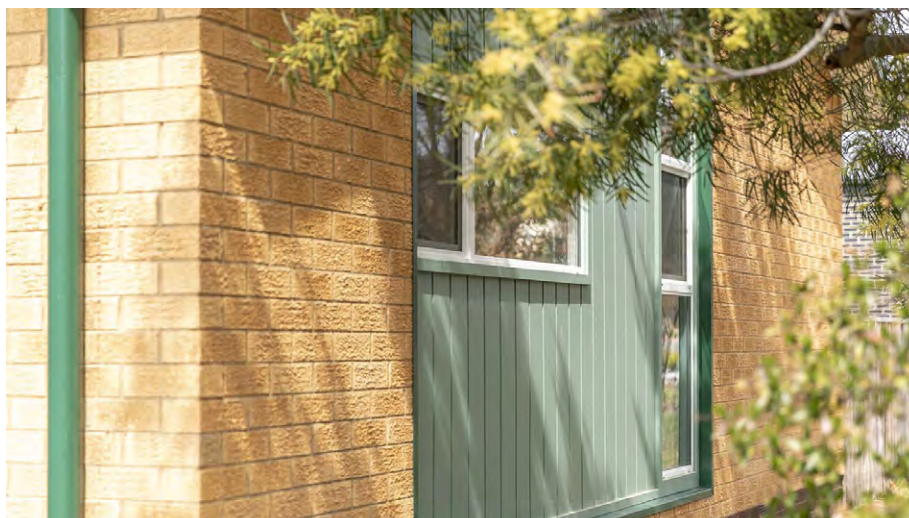
FIGURE 16 Reconfigured existing window SOURCE: Light House Architecture 'Fab-ode'
